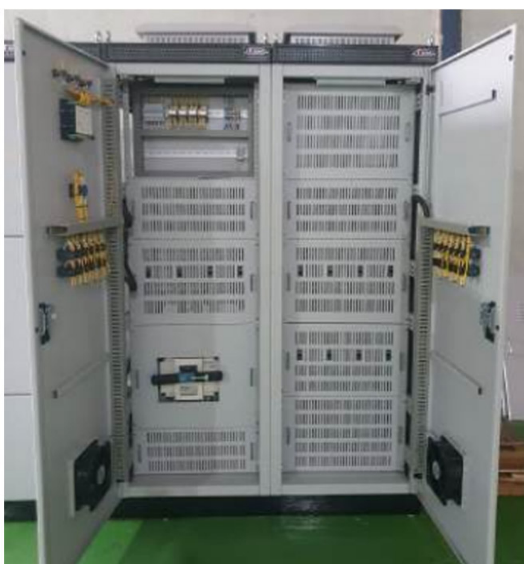
Panel Capasitor Bank – Project Factory Bogor
